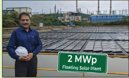
Floating Solar Power Plant
