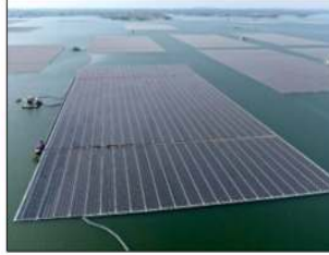
Worlds Largest Solar Floating Project (O&M) - Omkareshwar, Madhya Pradesh
